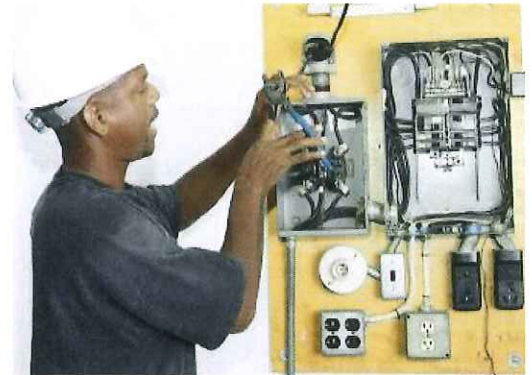
Electricians connect a variety of fixtures to internal and external electricity sources.
